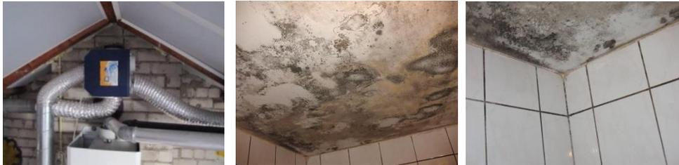
*moulds on bathroom ceiling; bathrooms in particular need proper ventilation*
