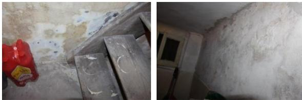
*moisture on cellar walls, often due to a lack of ventilation, regularly due to leaks*
