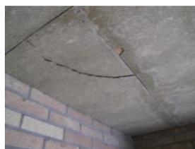
Garage ceiling containing asbestos
