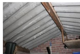
Storage room roof containing asbestos
