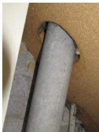
Ventilation shaft containing asbestos
